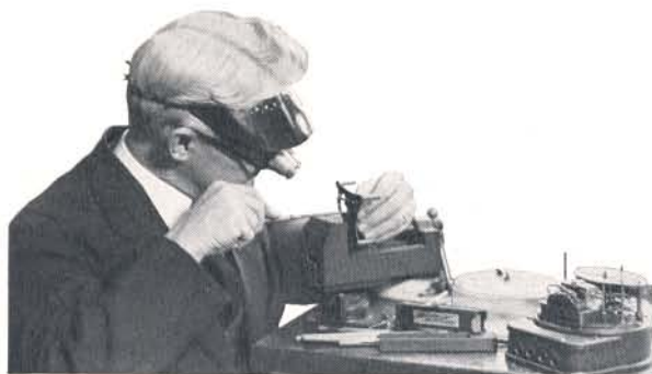
Filing a delicate part of an electric meter with an "American Swiss" needle file.
